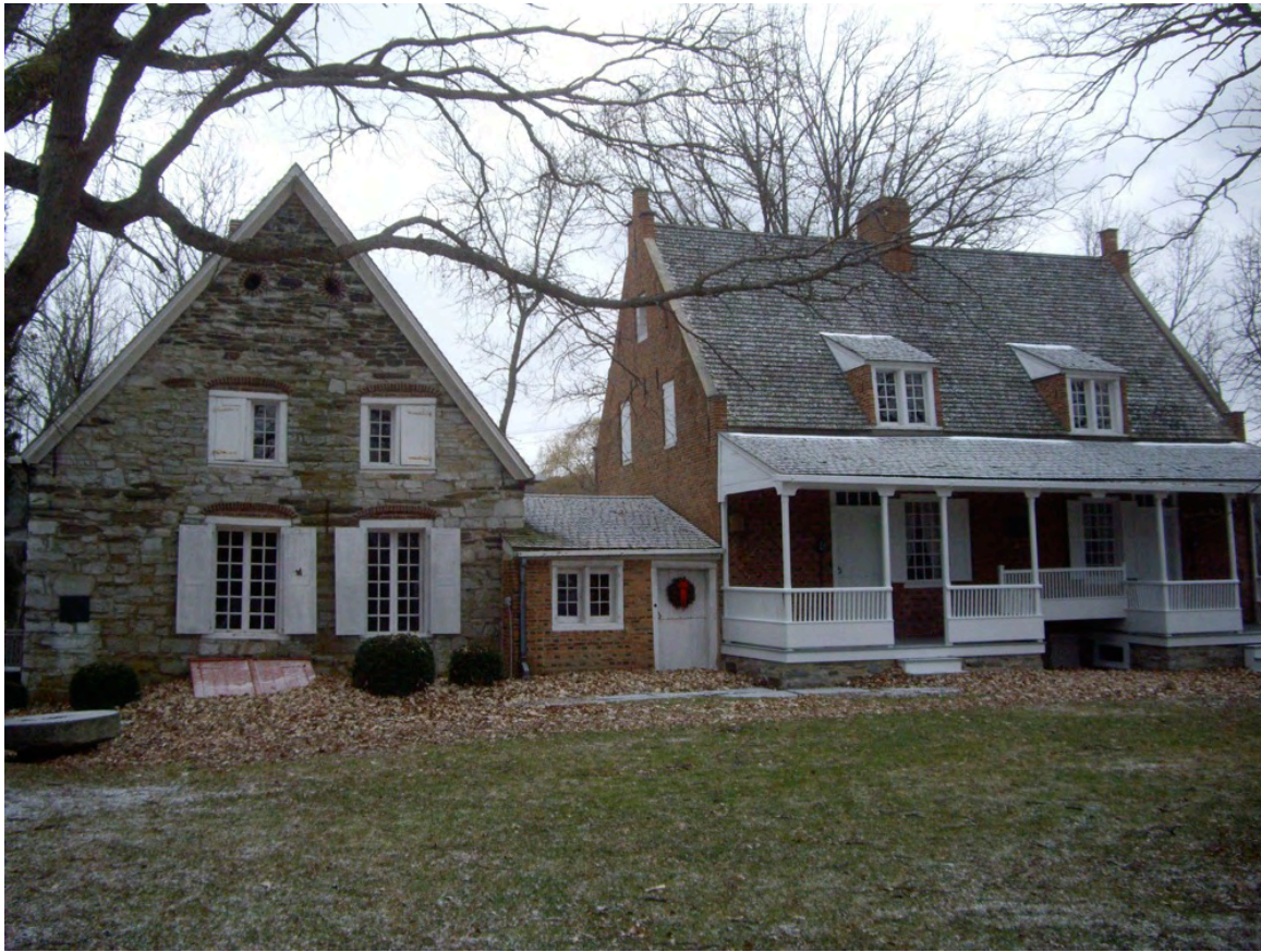
Peter Bronck House, Cossack, NY 1663 – original structural stone 1738 – H-Bent frame with brick veneer
