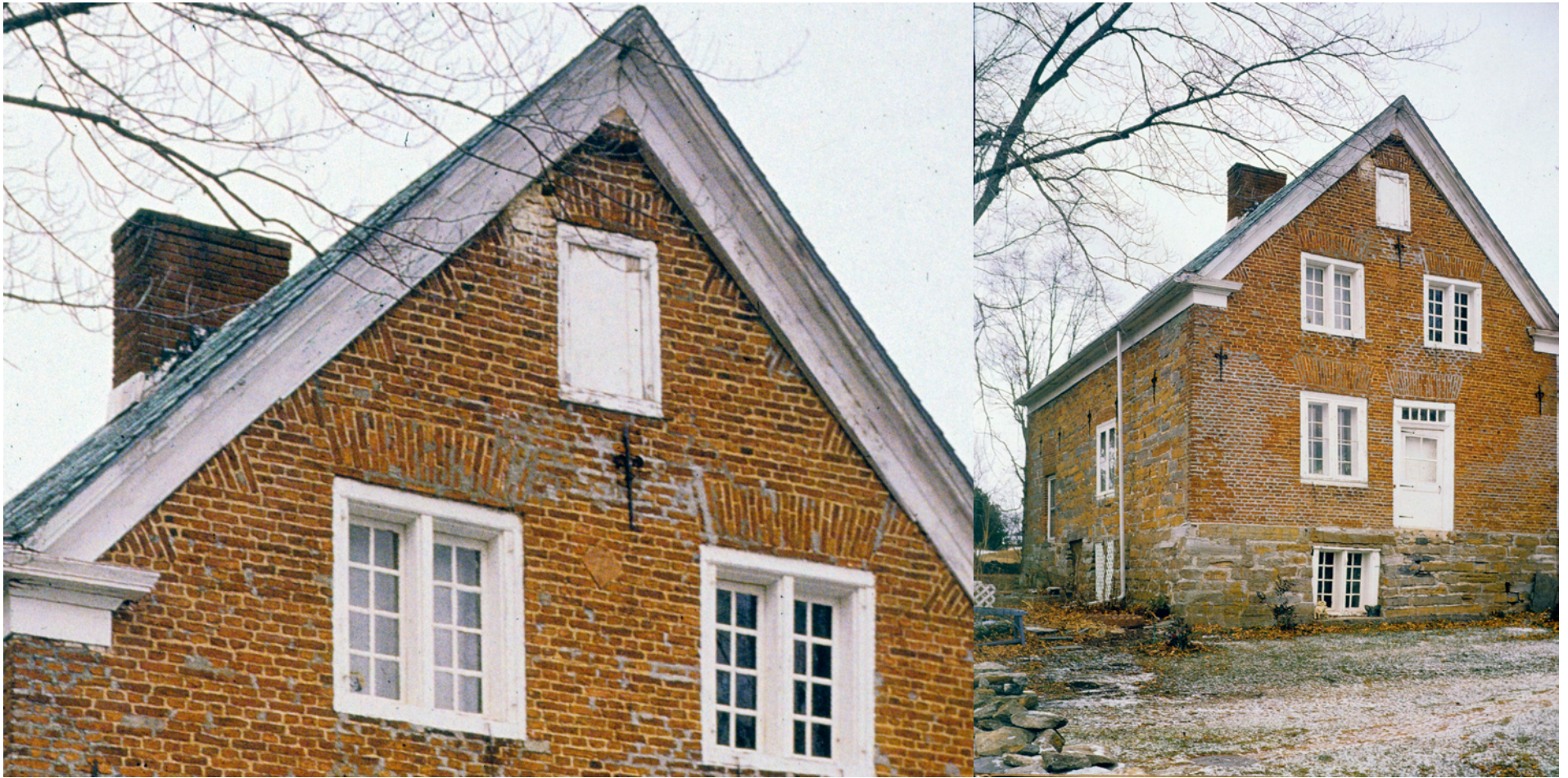
“Mousetooth Bond” on parapet gable, not stepped
